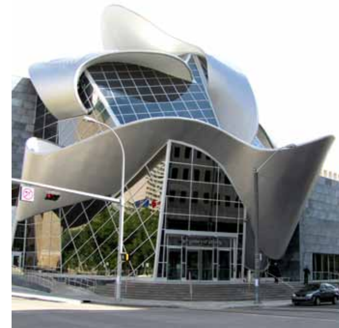
Art Gallery of Alberta, Main Entrance, 2010 Photograph Courtesy of Shane Golby
