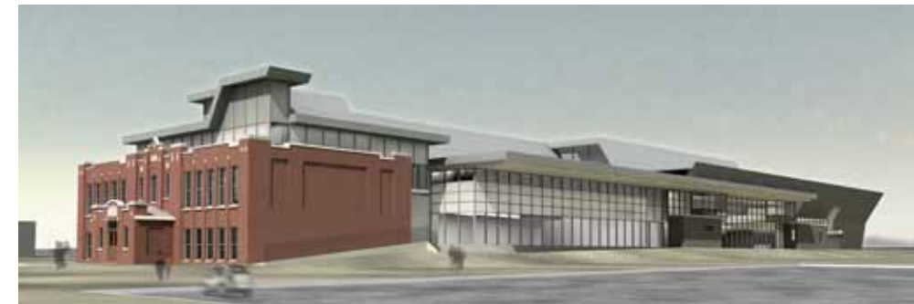
Prairie Art Gallery/Montrose Cultural Centre, Grande Prairie Artist Rendering Credit: Teeple Architects, Toronto Exhibition: Culture Crates
